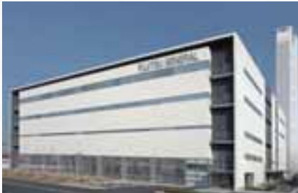
R&D Center And 60m Height Difference Testing Tower
